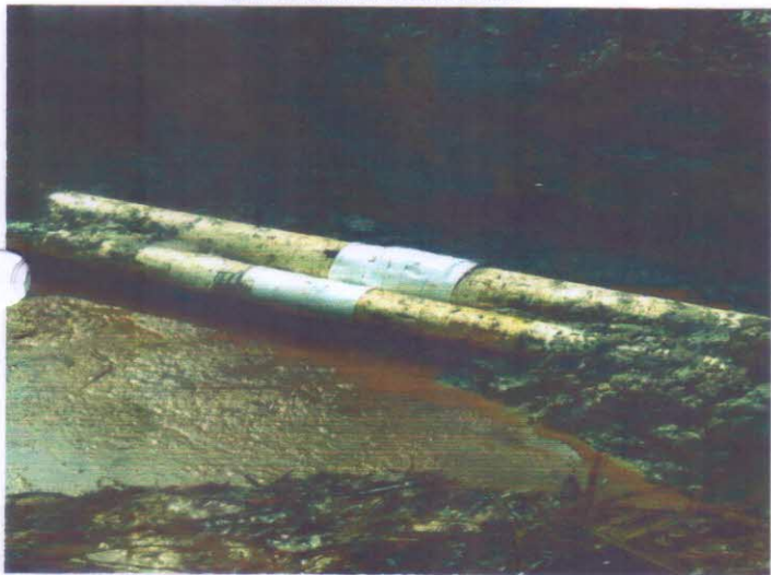
REPAIR WORK SHOWN
